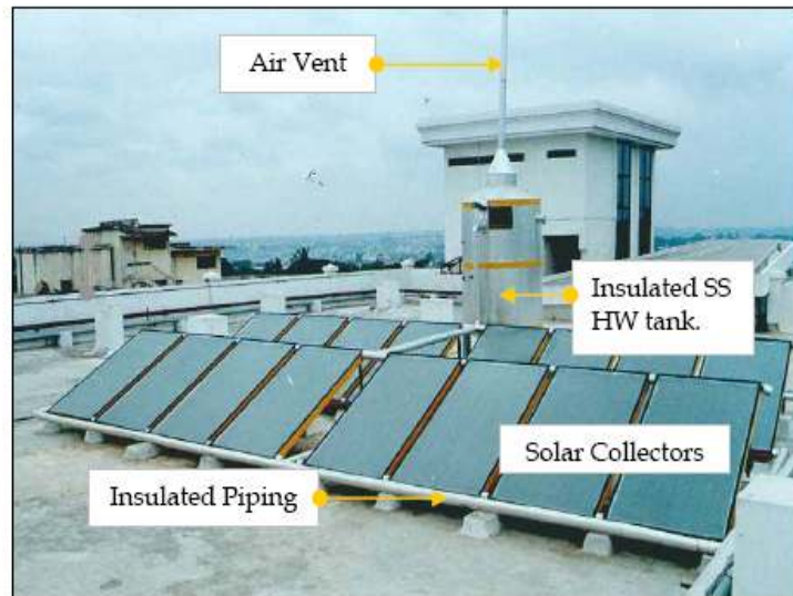
Typical 'Solar Water Heating System' (SWHS) components.
